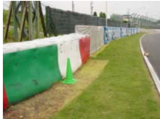
(Figure 2) Tire barrier and foam barrier (the green cone is a counterpart)
